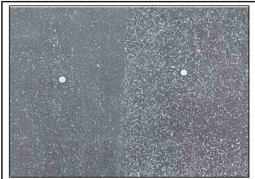
Photo B-4. Close-up view of Bleeding, High and Medium Severity High Severity on left shows most aggregates covered with asphalt and Medium Severity on right shows less aggregates covered with asphalt
