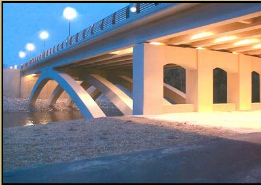
Siebenthaler Bridge, Montgomery County
