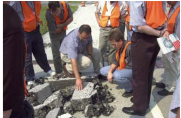
Site Visit to DEL-23 Test Section - Issam Khoury, OU
