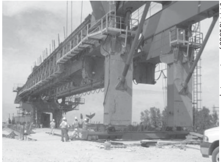
The erection trusses in normal operation prior to the tragedy.
