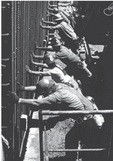
Workers secure re-bar on Boston's Big Dig Project. Image by Michael Hintilan from the Big Dig Web site.
